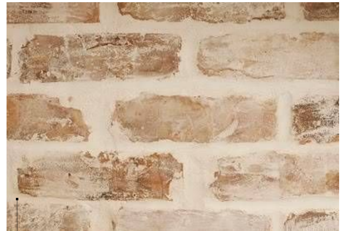
overfill grout joints to be flush with the brick face
